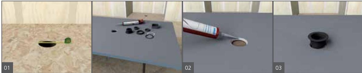
1. Cut the 2 in. (50.8 mm) pipe flush (or max. 1/8 in. [3.2 mm] above) to the floor construction. Make sure that the cut out fits to the Fundo panel drain. Cut out a 5 in. (127 mm) diameter hole around the 2 in. (50.8 mm) pipe to allow for the wedi drain to be inserted into the subfloor while the cut out area must remain free of deflection. Sturdily fasten the drain and trap to the subfloor. Assemble the drain unit following the instruction drawing.
