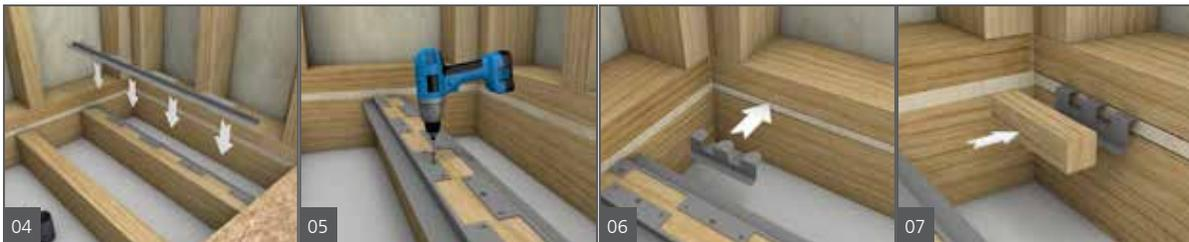
4. Fasten the next bracket on the other side of the floor joist. The mounting tabs must be staggered from those on the first bracket; this may require cutting the second bracket.
