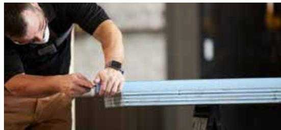
A wedi shower base can be cut to size using a circular saw with standard carbide blade. You can remake the 1/2 in. x 1/2 in. perimeter channel by cutting through the cement surface using the circular saw set to cut 1/2 in. deep. You can use a circular saw or a sharp utility knife to cut the new channel 1/2 in. wide through the blue exposed foam side. Clean the new channel and the base and remove all saw dust and loose particles.
