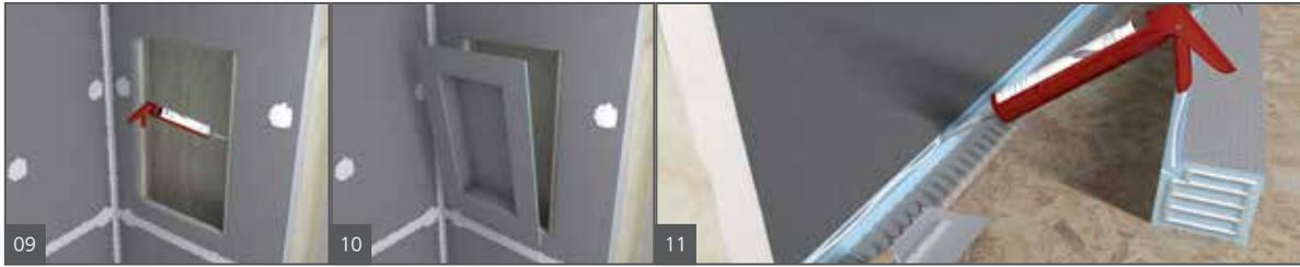
9. wedi Niches are installed in a cutout in the building panel and attached with its flange right into the center of 16 in. (406.4 mm) o.c. studs. Use wedi Joint Sealant along the connection of the wall to the niche. Use two fasteners on each side, keep in mind larger niches require more than two fasteners on each side, of the niche to create a flush transition to the wall panels. Another 1/2 in. (12.7 mm) bead of wedi Joint Sealant must then be spread over the fasteners and seams.
