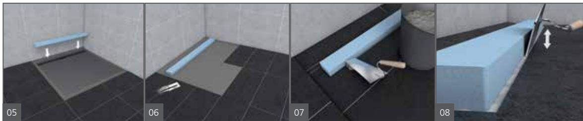
05 Use the foam block (provided) as a spacer for thinset mortar.
