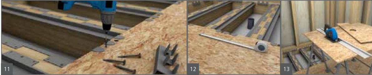
11. Use the shorter Phillips head self-drilling screws with wings provided by wedi to fasten C brackets to the edge of the wood subfloor at the open side of the shower area. Fit the brackets between flanges of the joist/wall brackets. Use two screws to fasten this bracket through the wood floor and into the lower claws.
