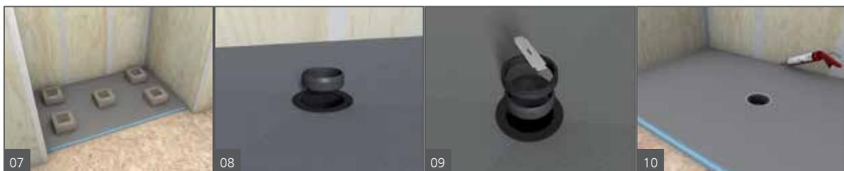
7. Press the Fundo firmly into the thinset bed, ensuring that the installation is level and void free. Apply some weight equally on top of the base. Leave on the surface and drain area to allow the thinset to initially cure without being disturbed (e.g. tile boxes).
