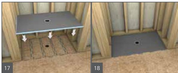
17. Install the wedi Fundo Ligno shower base in a bed of tile adhesive as per the Ligno installation manual.
