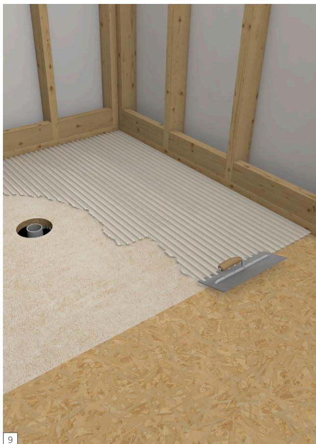
**EN** Clean the subfloor with a moist sponge to remove dust and dirt, and apply a skimcoat of a suitable, modified tile adhesive/ thinset (ANSI 118.4 or better), and comb through with a 1/4 in. × 1/4 in. notched trowel. Notches should be applied uniformly and point towards the shortest side of the base area. You can also use a 1/2 in. square notch trowel, instead.
