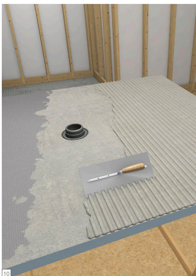
**EN** Trowel the thinset on the rear side of the Fundo again using a 1/4 in. × 1/4 in. notched trowel. Apply a skimcoat of tile adhesive over the entire product's cement surface, then comb through thinset bed creating channels pointing in same direction as applied on subfloor.
