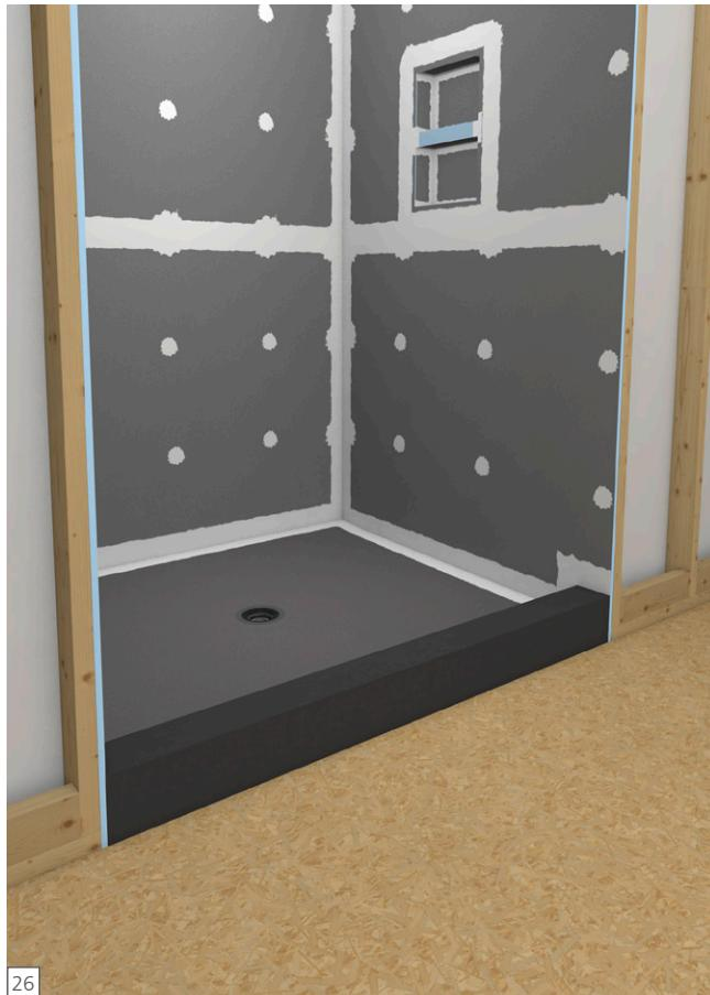
**[EN]** Weight is applied for a minimum of 30 minutes on and against the curb (from outside) and another 1/2 in. bead of sealant is applied over all curb seams and spread flat. The seams must be covered 1 in. either side of a seam.
