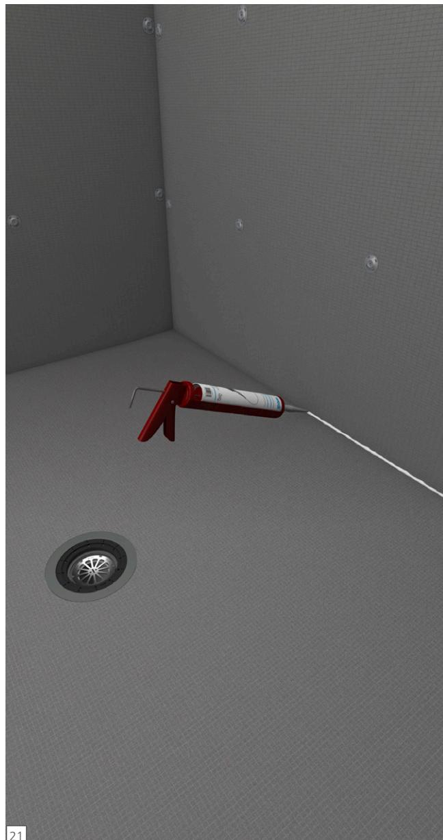
**EN** Apply continuous 1/2 in. beads of sealant between all connections of panels and install with tightly butted seams. Excess sealant must be spread flat with a putty knife. All seams and fastener heads in the assembly are covered with a topical 1/2 inch bead of sealant and spread flat. The seams should be covered 1 in. on either side of a seam. All fastener/washers are covered with sealant stretching 1 in. over the washer edges.
