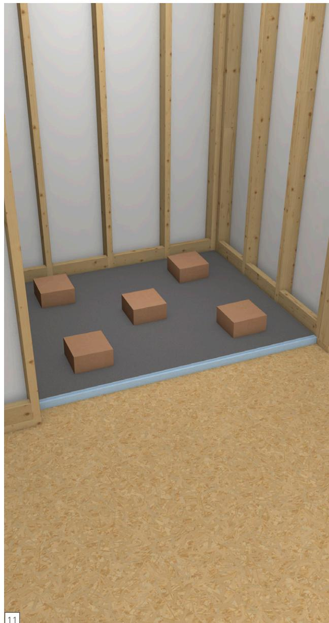
**EN** Press the Fundo firmly into the thinset bed (sloped side up) ensuring that the installation is level along its perimeter and sides, and thinset attachment and coverage is void free. Apply some weight equally and leave on surface and drain area to allow the thinset to initially cure without being disturbed (e.g. tile boxes). Make sure the floor waste pipe is centered within the wedi drain unit and remains there until the drain connection is completed.
