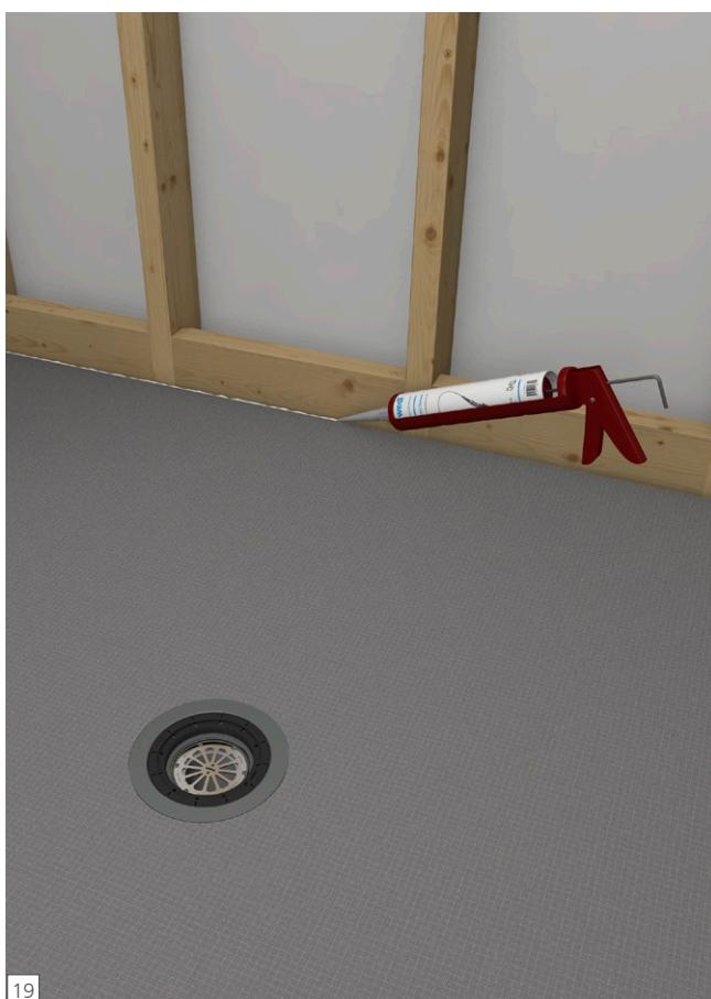
**EN** Dry fit the building panels to ensure the proper fit into the perimeter channel. Clean the perimeter channels from dust or any other contaminants. Set up a continuous 1/2 in. bead of wedi Joint Sealant along the Primo's channel on the outer perimeter and only in areas where you can immediately install a building panel into the fresh sealant.
